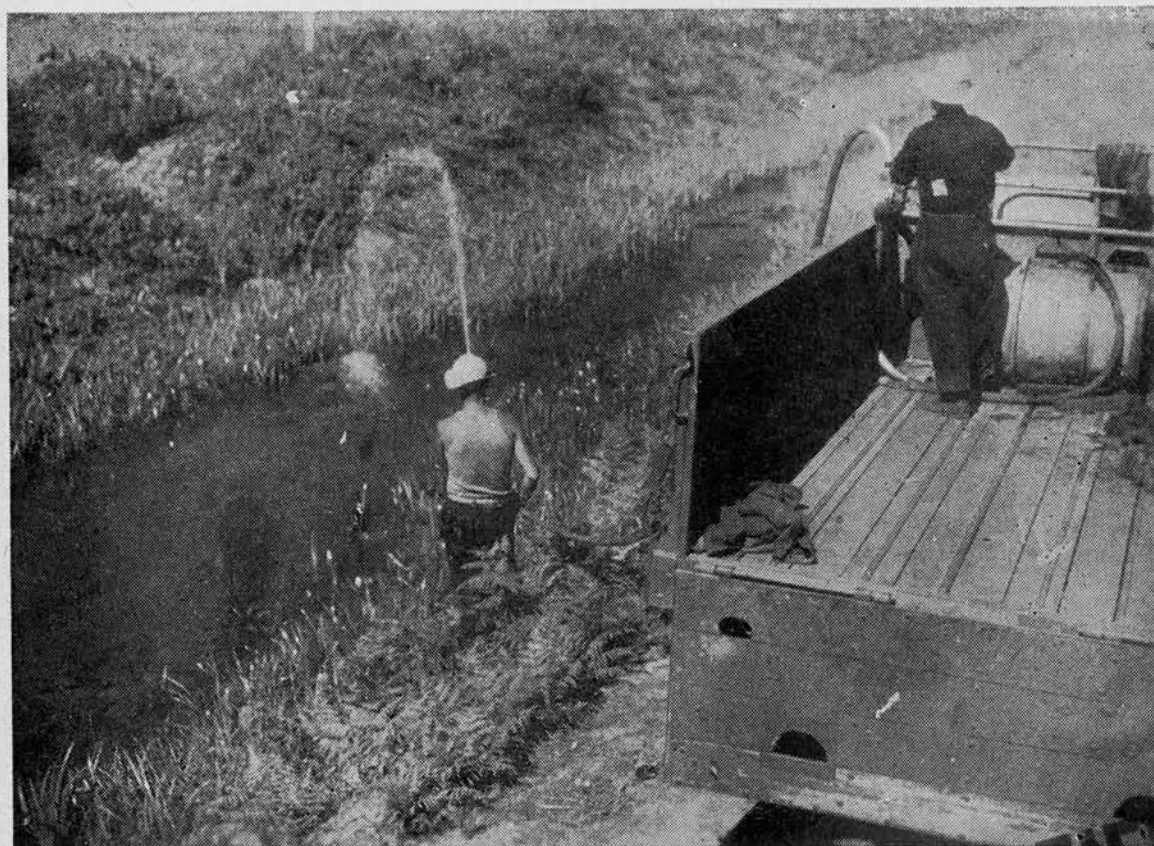
Oiling with a converted petrol pump at Alto.
